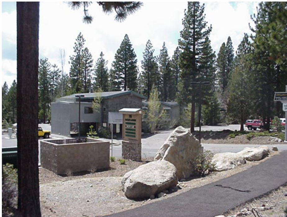
The Incline Creek Commercial Building.
